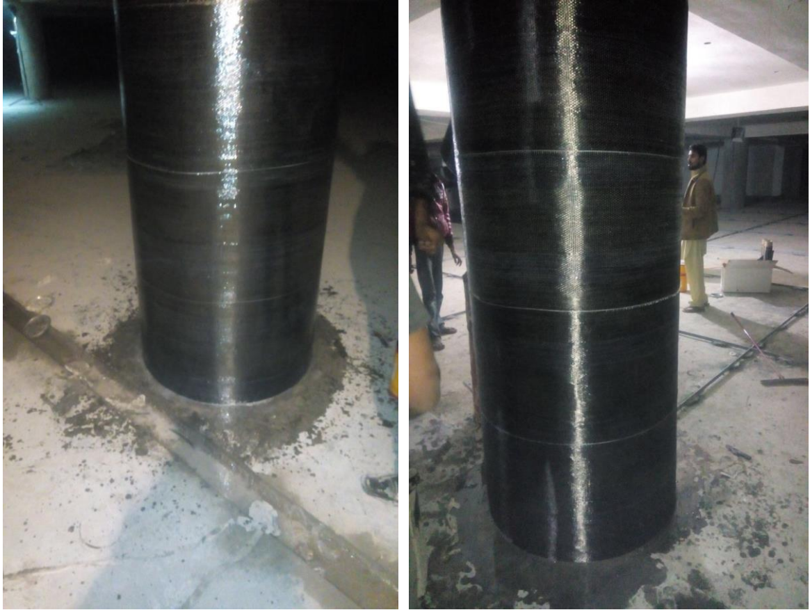
Final look of Column Strengthening at Amanah Mall, Lahore
