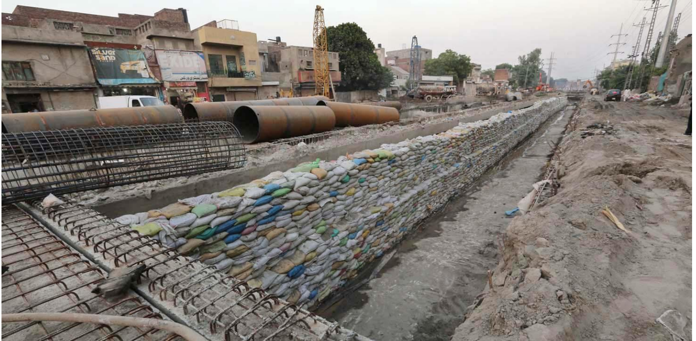
LOS Drain under Construction
