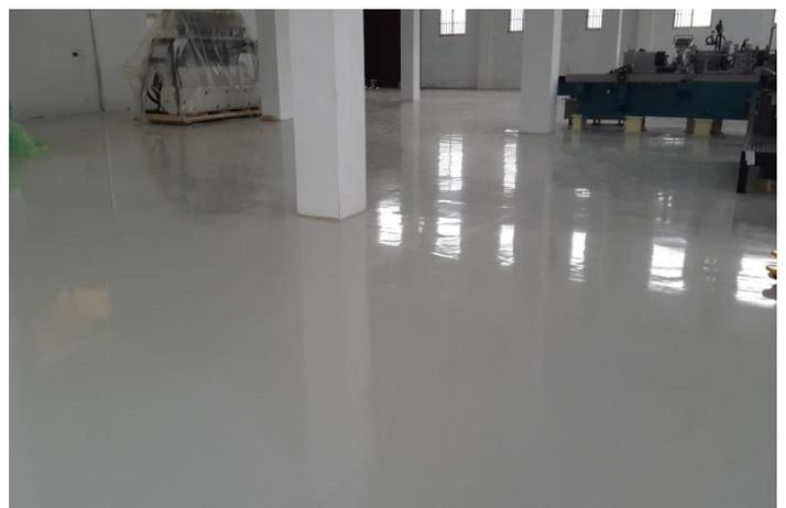
Sikafloor-264 is used as a Roller coat for concrete and cement screeds with normal to medium heavy wear e.g. storage and assembly halls, maintenance workshops, garages, loading ramps and car parks maintenance hangars and for wet process areas, e.g. beverage and food industry. Sikafloor-264 is an environmentally friendly solution that also, provides Good chemical and mechanical resistance.
