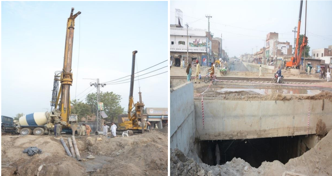
Above are some pictures of Gujranwala Underpass Under Construction
