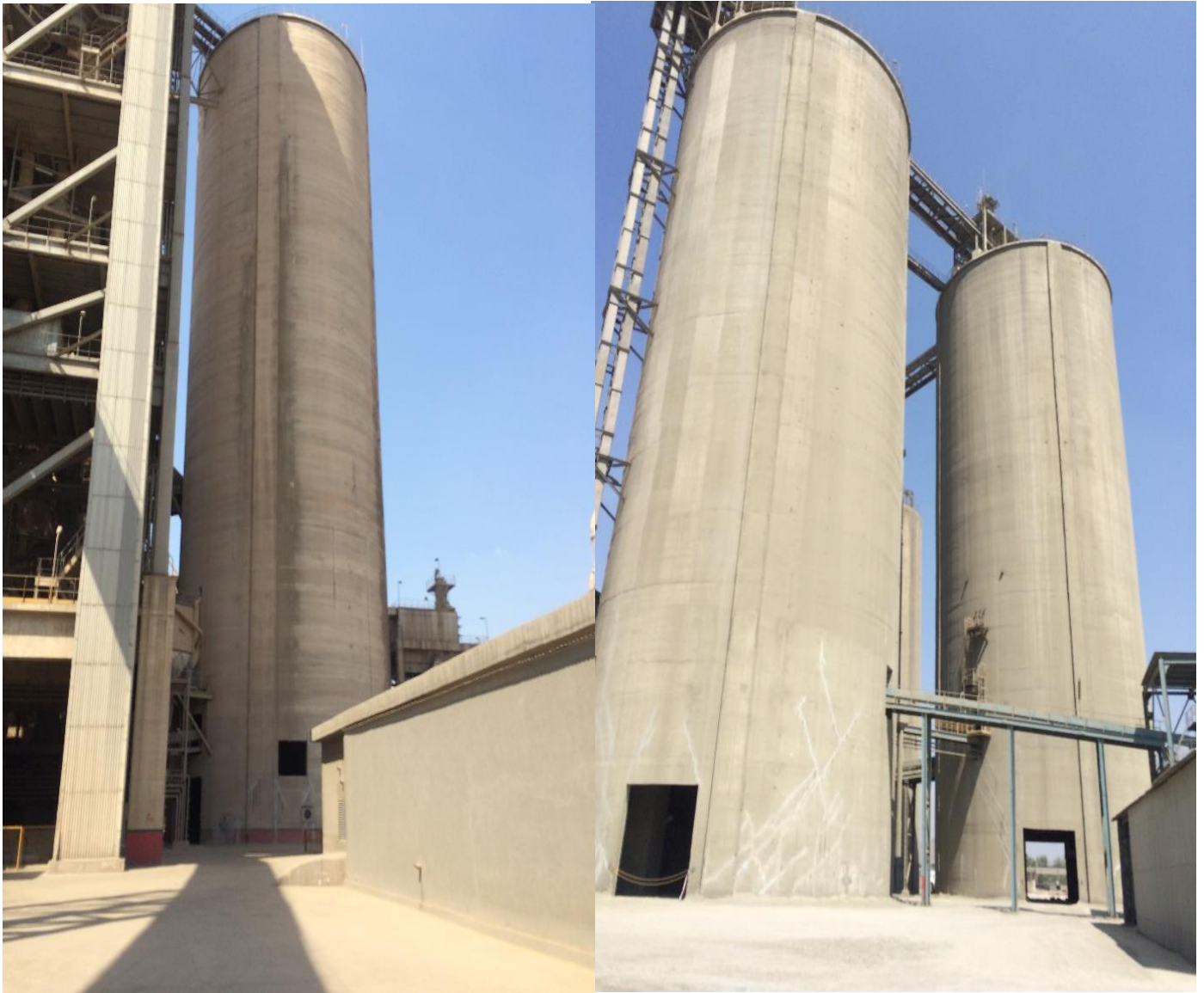
Final look of Silos after the application of Sika CarboDur ® structural strengthening system
