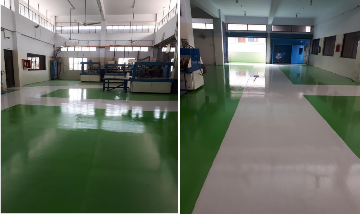
Final look of Flooring at Phoenix Battery Production Facility, Karachi
