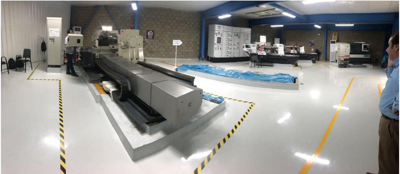
Final look of Flooring at Amreli Steel Production Unit CNC Room, Dhabeji Karachi
