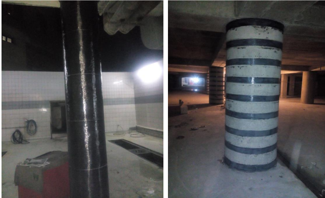
Final look of Columns after the application of SikaWrap-230 C at Honda Fort Showroom, Lahore
