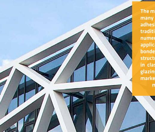
The modern way of installation for many things is with elastic adhesives. Compared with traditional methods there are numerous advantages in both the application and life-cycle of bonded materials. Sika's silicone structural adhesives have the best in class ETA approved structural glazing design strength on the market, resulting in a reduction in material and sight lines.
